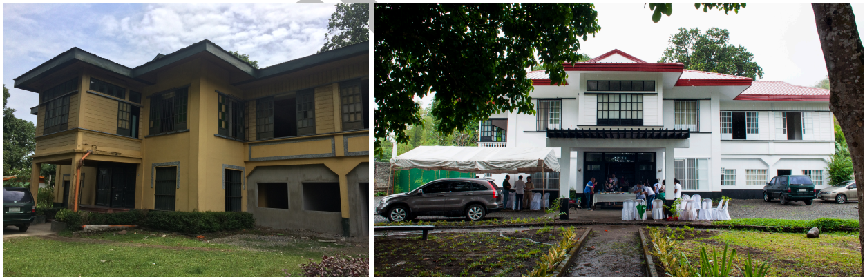
Figures 17-18: Before and after renovation of La Castellana house showing exterior
